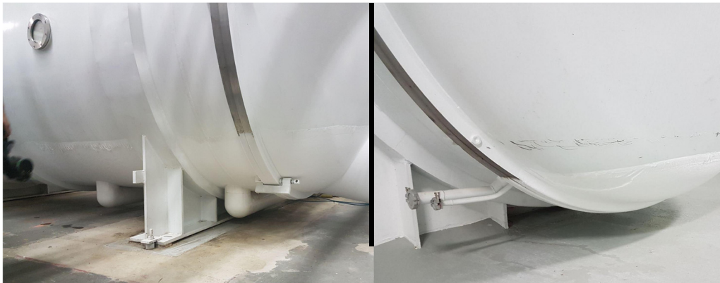
Figure 5: Ammonia frost line in the freeze dryer after the release.
