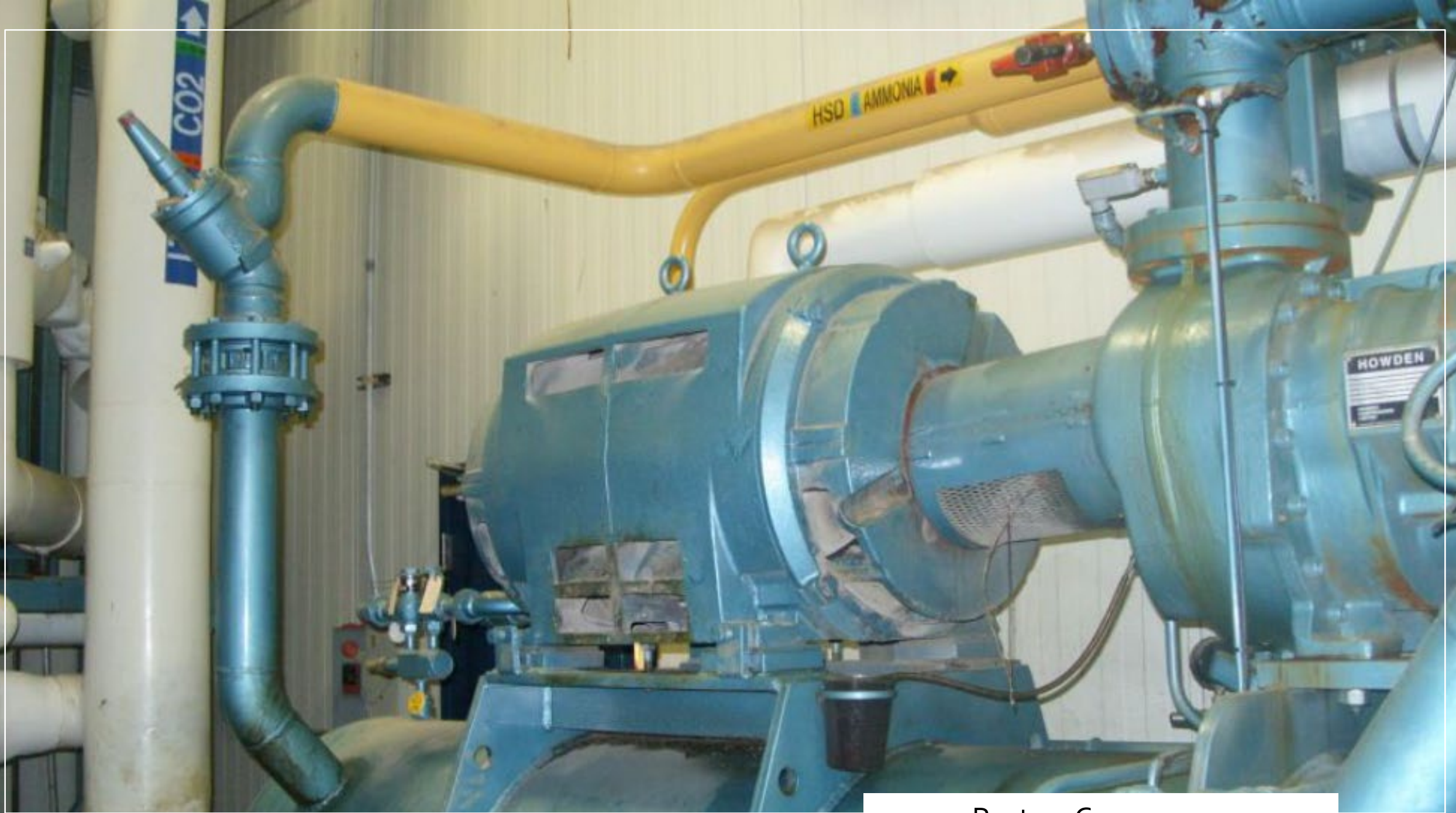
Rust on Compressor
