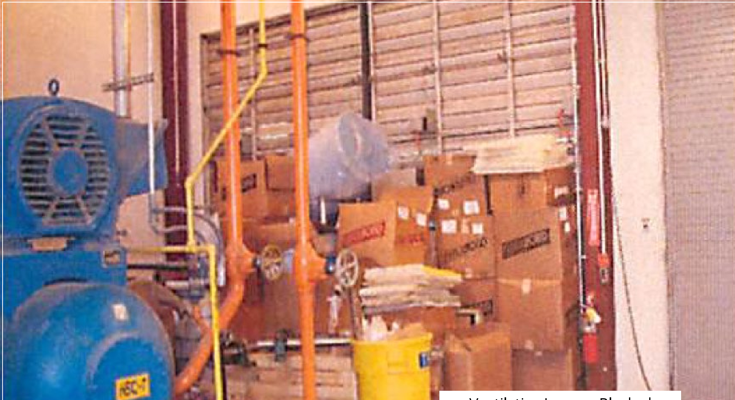
Ventilation Louvers Blocked
